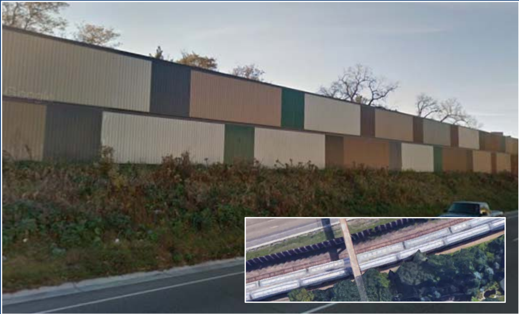
I-94 "Shipping Container" Noise barrier, Minneapolis, MN
