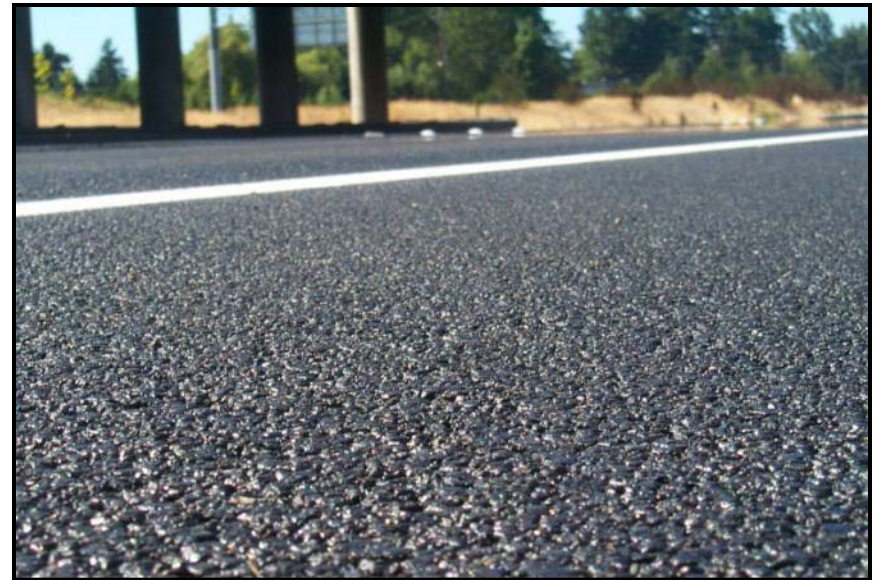
Newly installed OGFC-AR on I-5 (2006)
