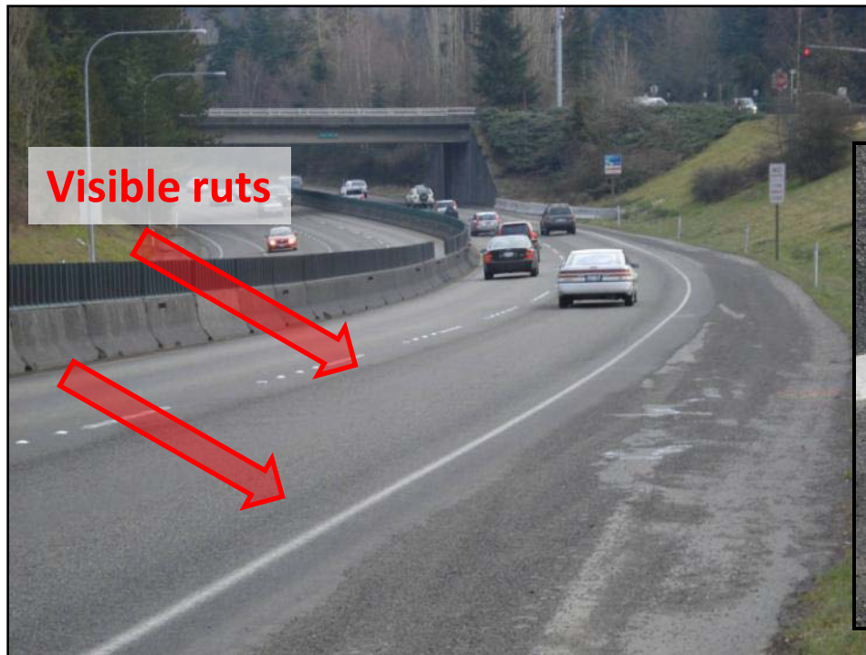
Raveled pavement and visible rutting on SR 520 OGFC-AR test section
