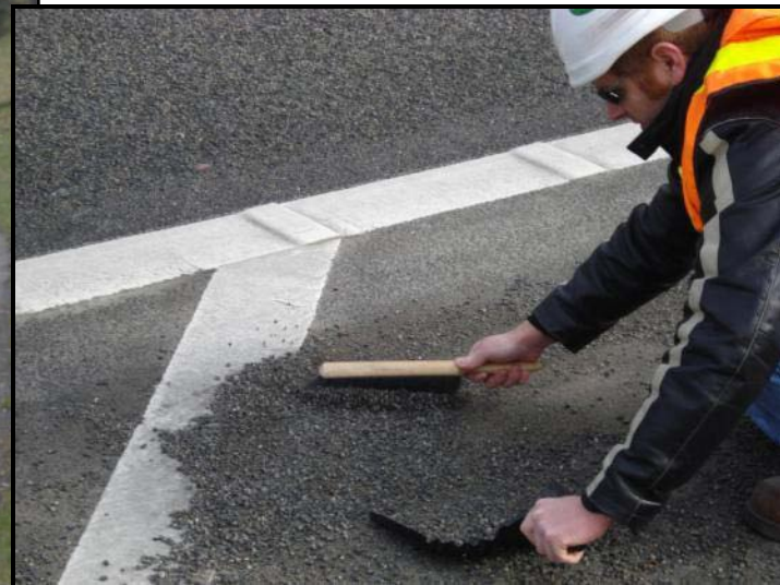
Raveled pavement and visible rutting on SR 520 OGFC-AR test section
