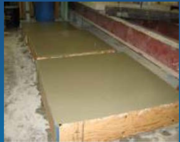
Finished PCC Slabs
